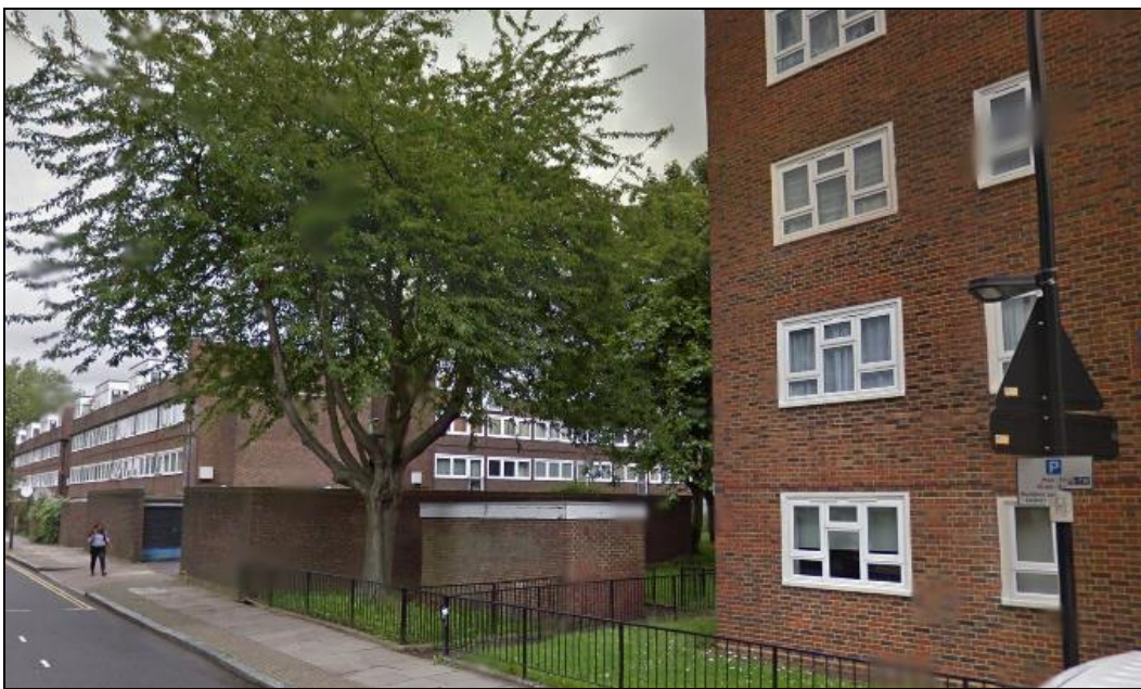
Image 3: View from the corner with Bavaria Road looking NW towards application site with 1 – 16 Cottenham Hose on corner
