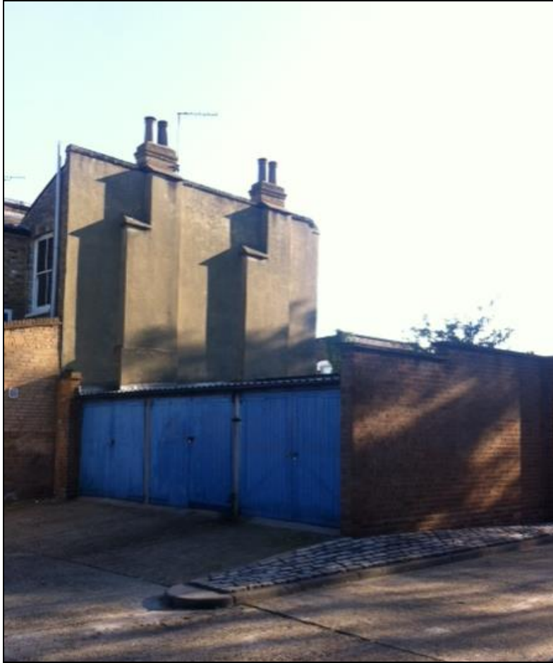
Photo 4: Existing garages to the front of the site
