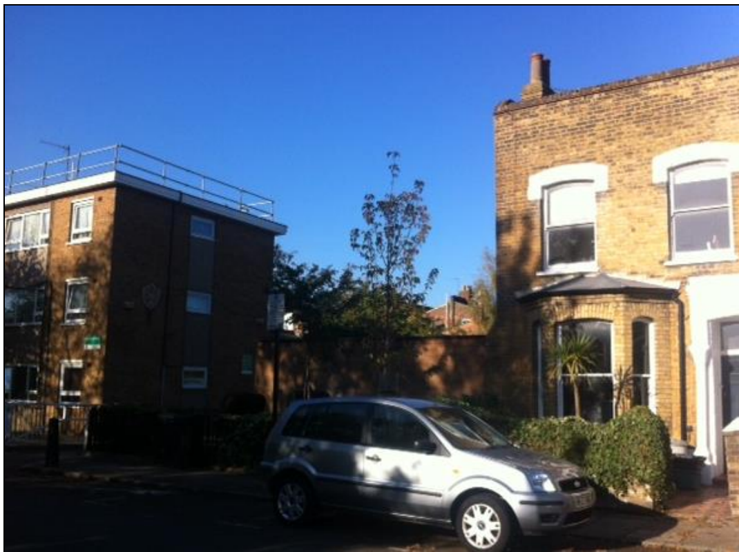
Photo 3: View of site from the north east
