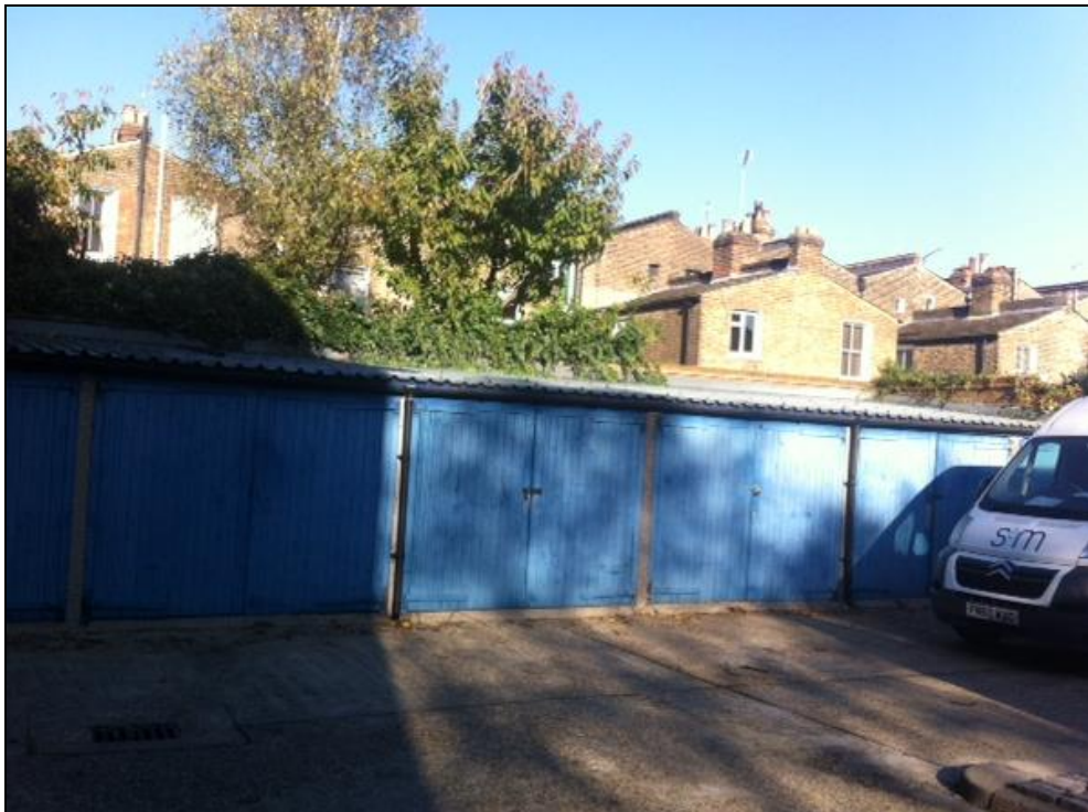
Photo 5: Rear garages to be demolished
